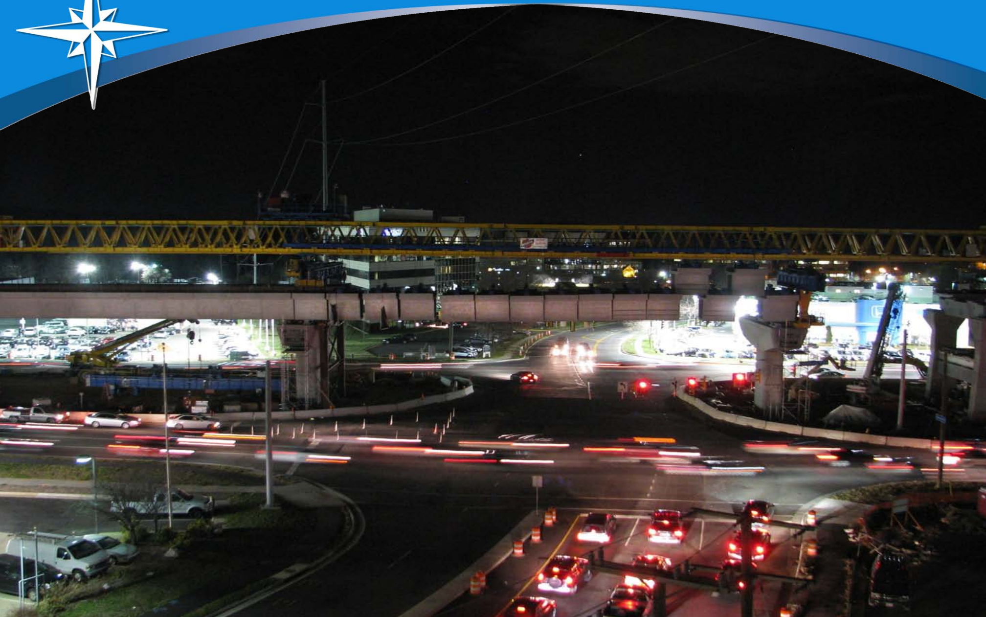
Spring Hill Road Guideway Crossing
