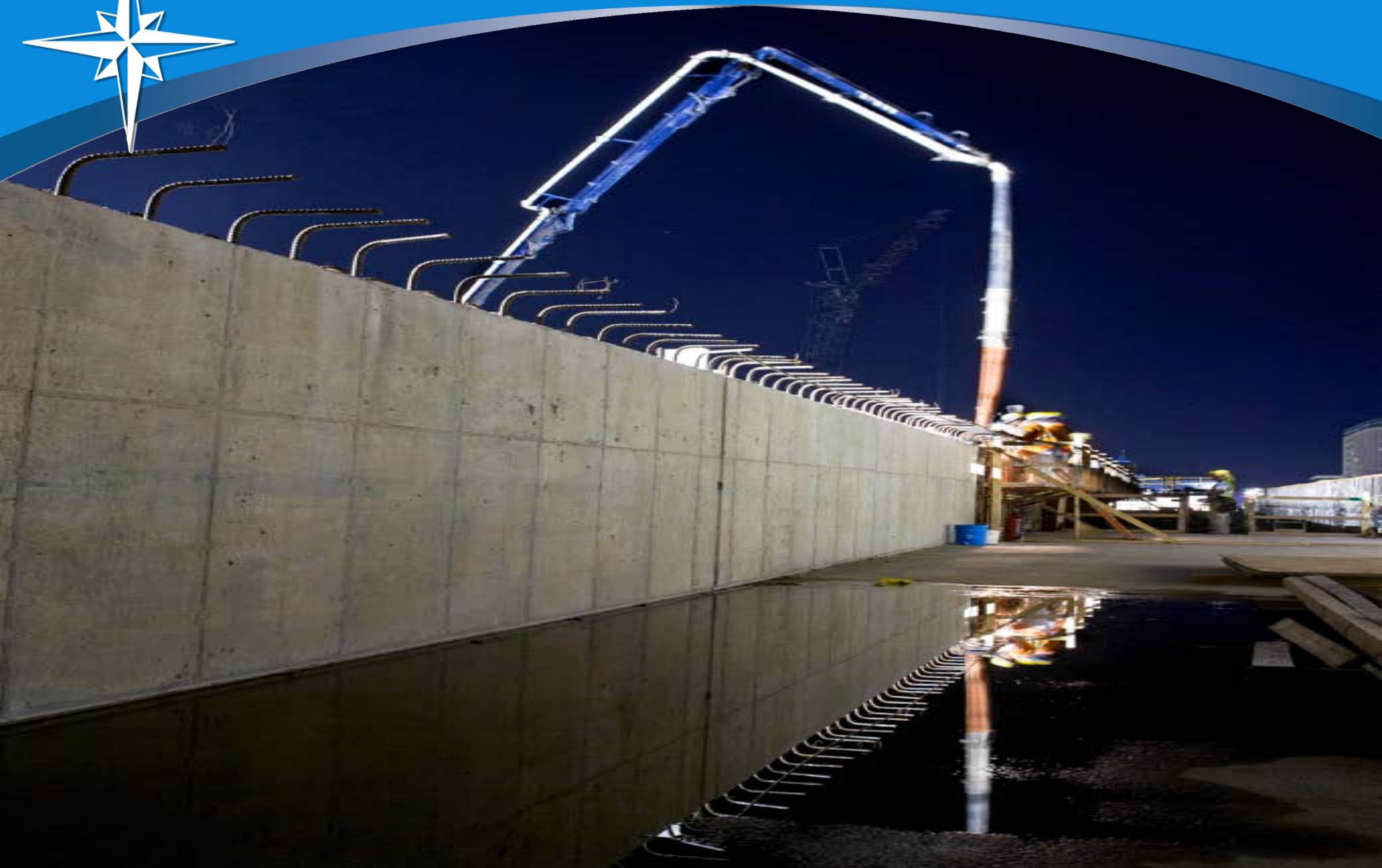
Station Retaining Wall
