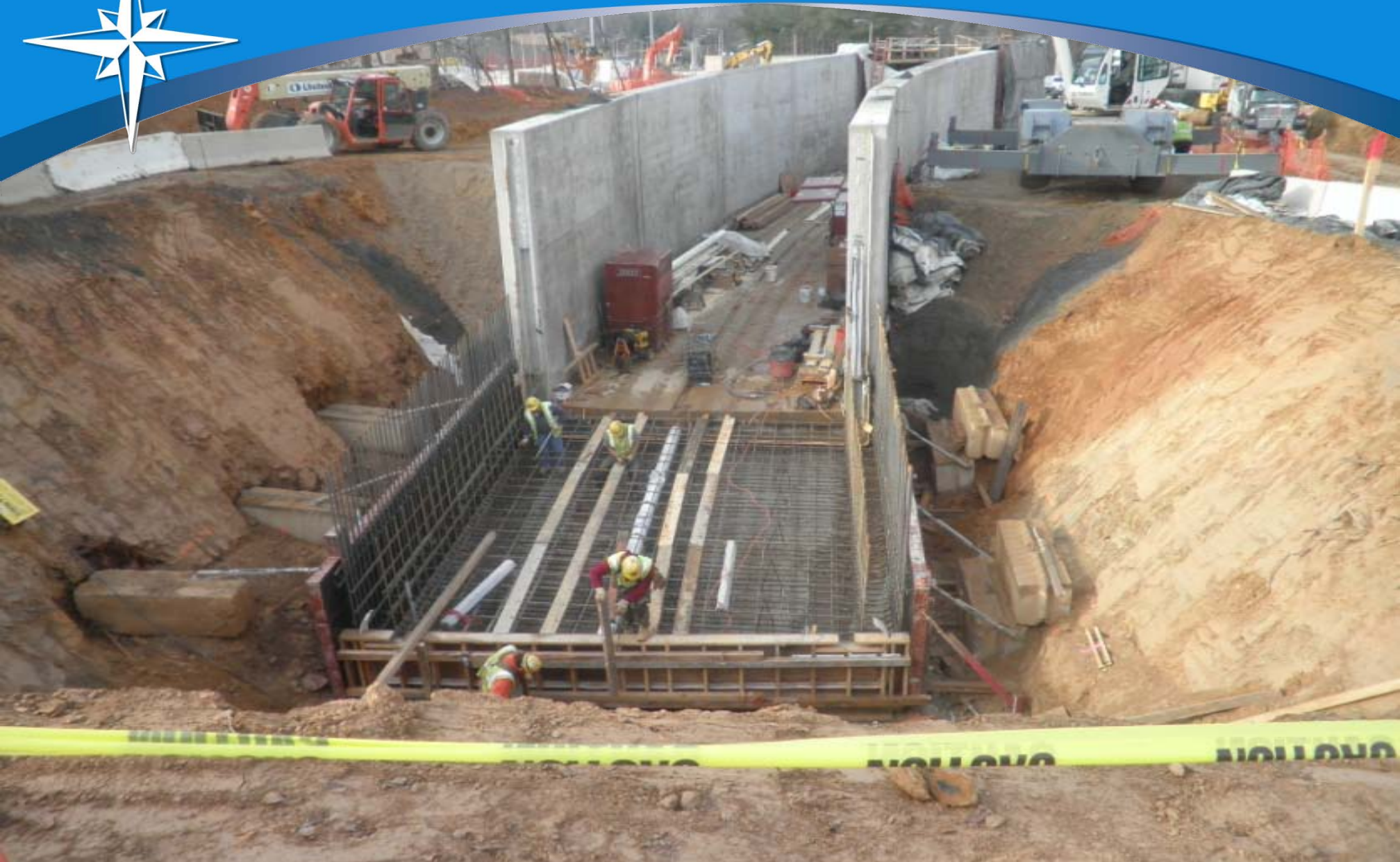
West Falls Church Yard Lead Track Tunnel
