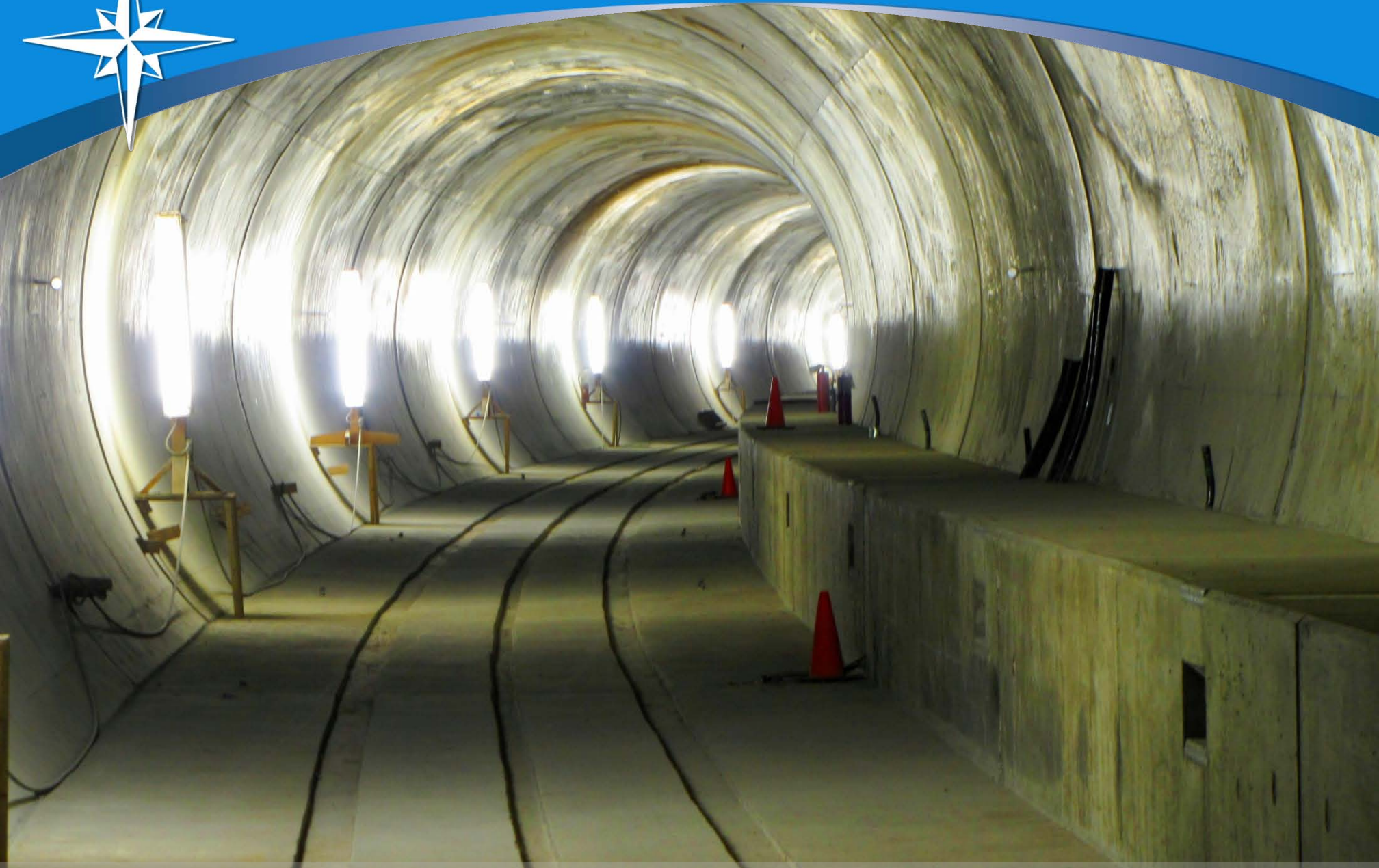
Tunnels at Route 123 and Route 7
