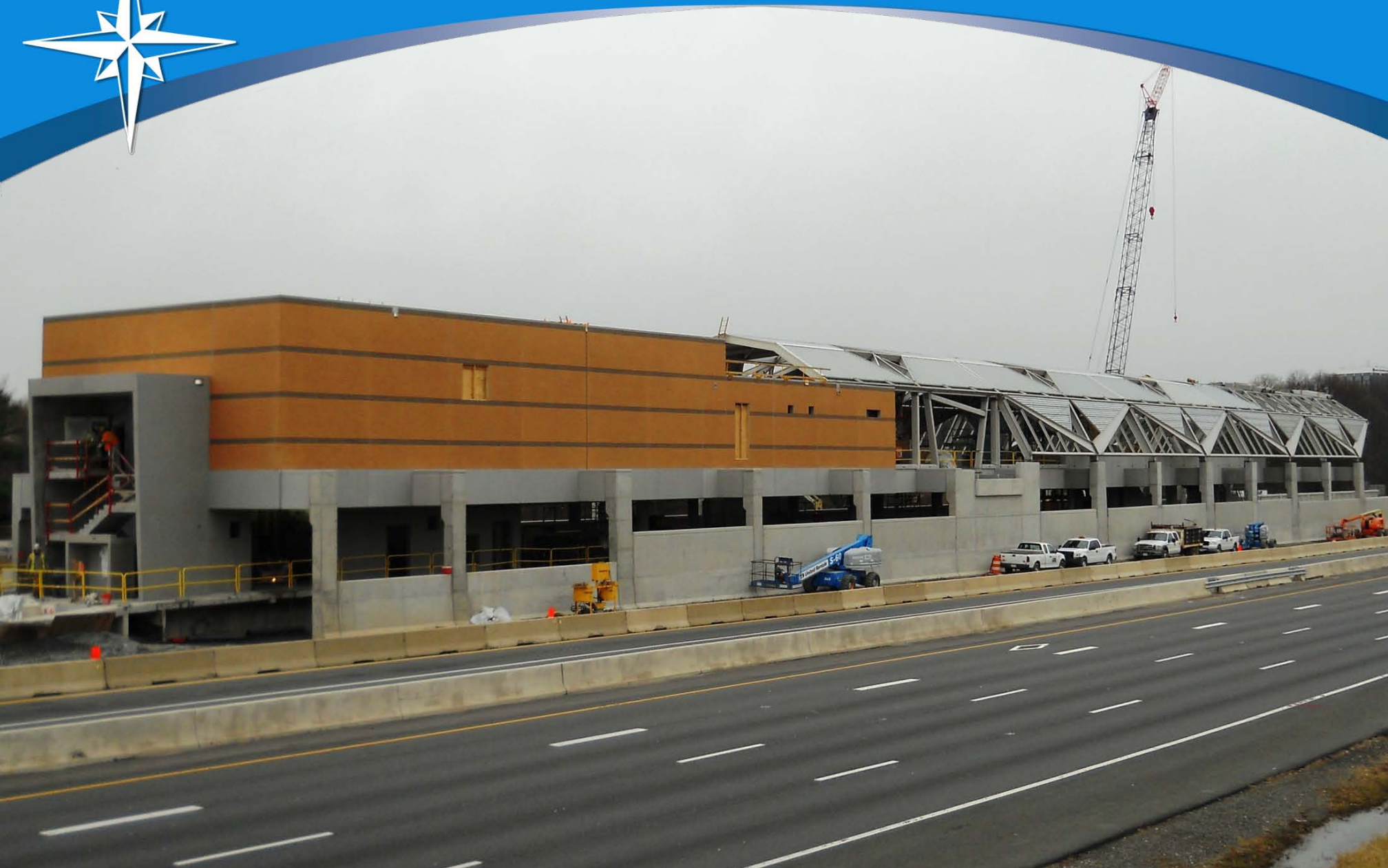
Wiehle Avenue Station
