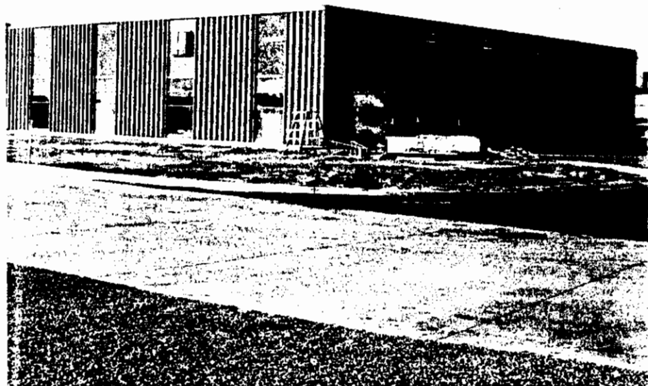
Plate 27 Allied Fuel Building
