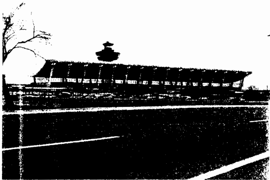
Plate 15 View of Main Terminal from Dulles Access Road at Main Parking Lot: View from the North
