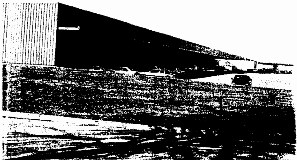
Plate 22 Cargo Building (Cargo Building No.1)
