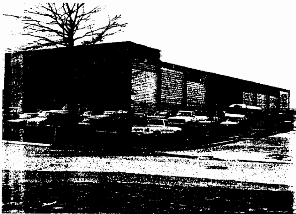
Plate 19 Vehicle Maintenance Building
