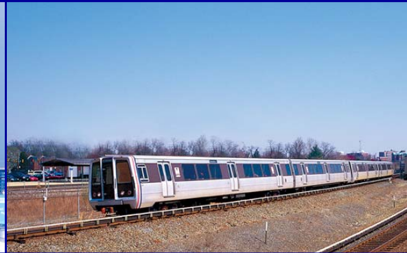
Dulles Corridor Metrorail Project
