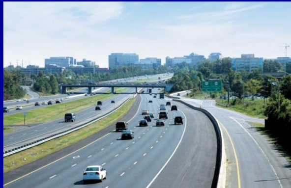
Dulles Toll Road
