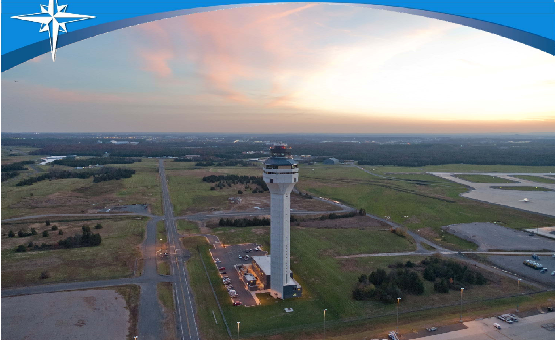
Airport Traffic Control Tower
