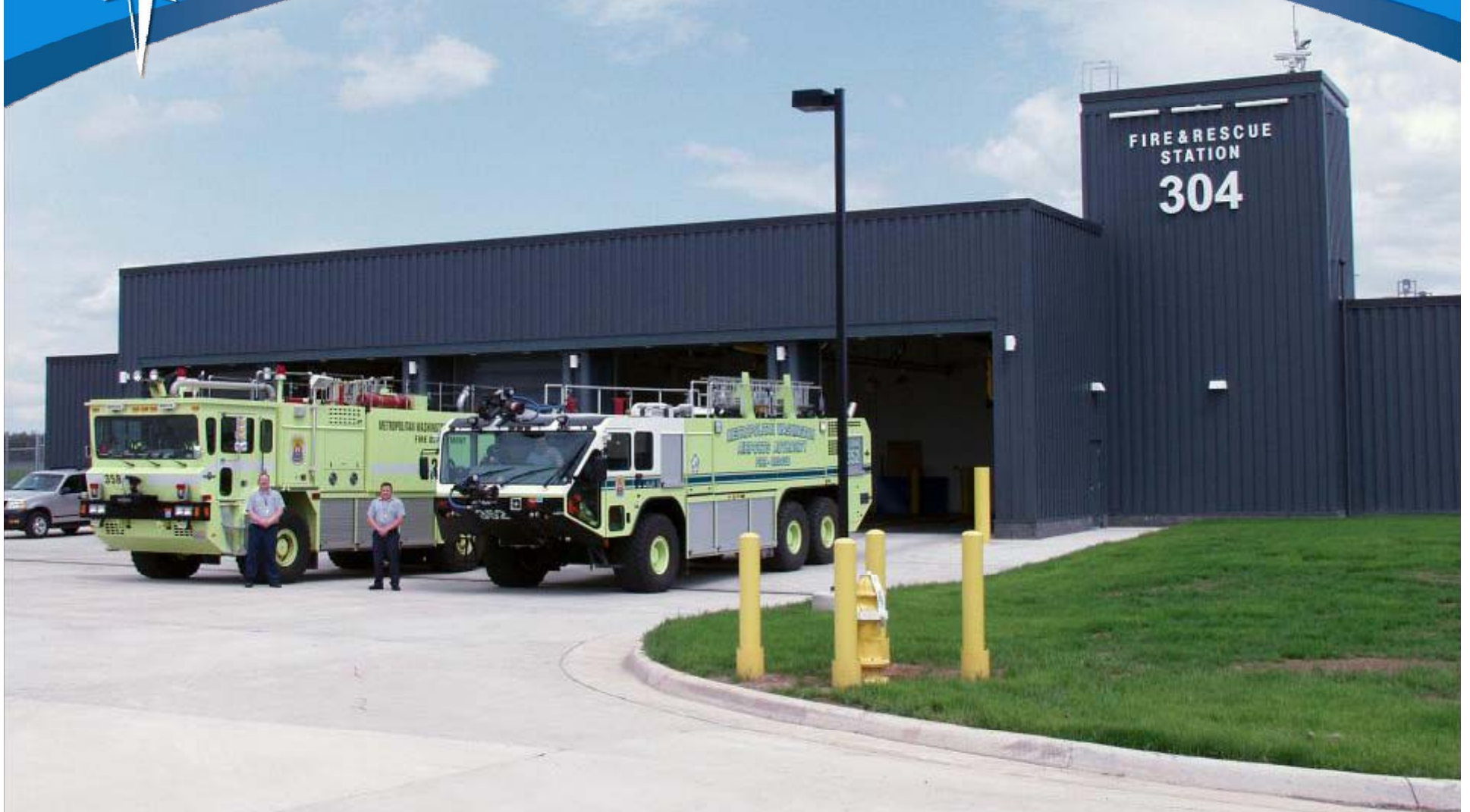
Airport Rescue and Fire Fighting Station 304
