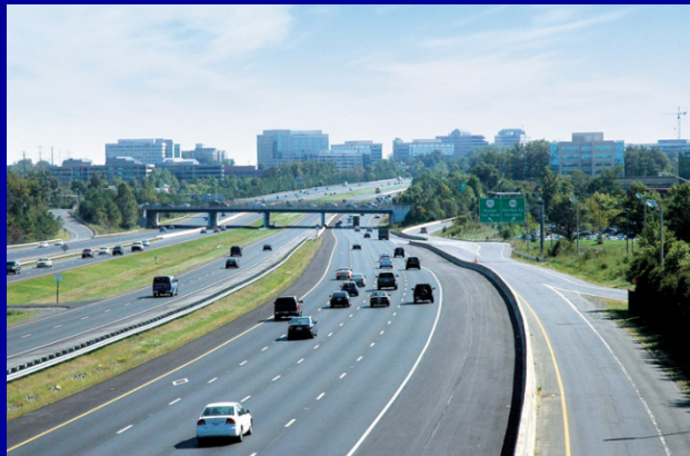
Dulles Toll Road
