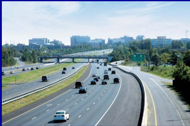
Dulles Toll Road
