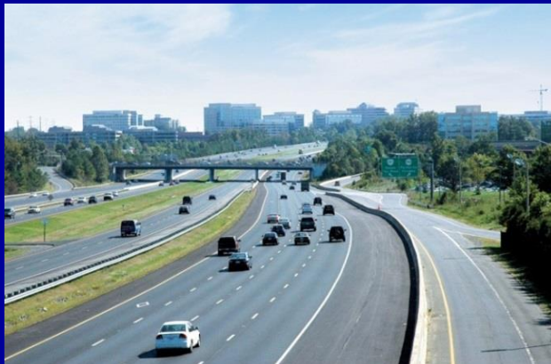
Dulles Toll Road
