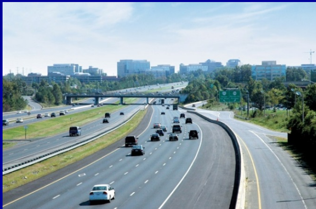
Dulles Toll Road
