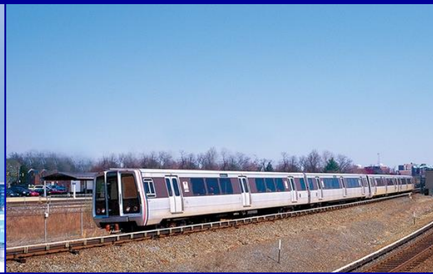
Dulles Corridor Metrorail Project
