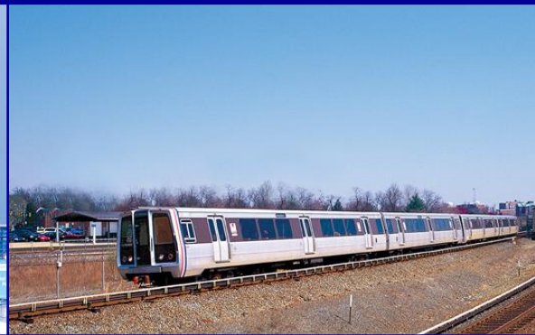
Dulles Corridor Metrorail Project
