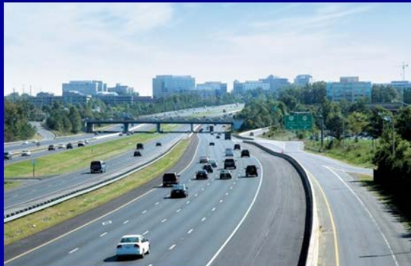
Dulles Toll Road
