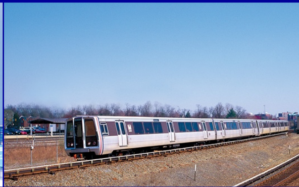
Dulles Corridor Metrorail Project
