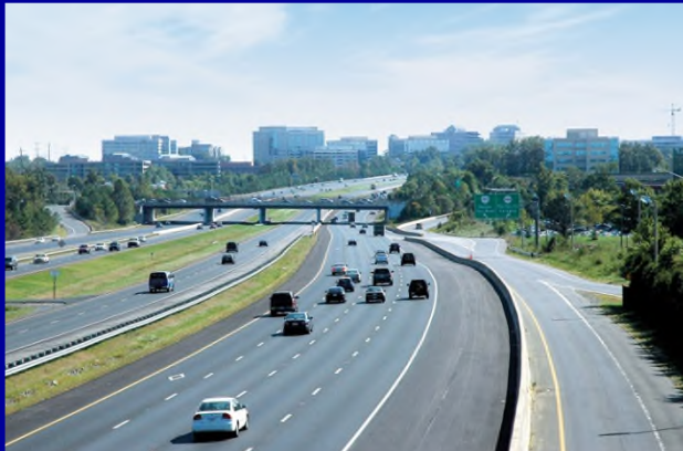
Dulles Toll Road
