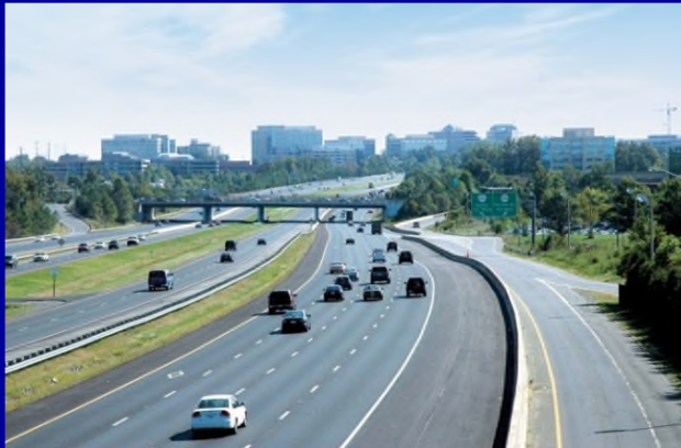
Dulles Toll Road
