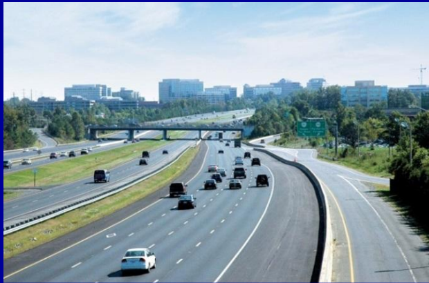
Dulles Toll Road
