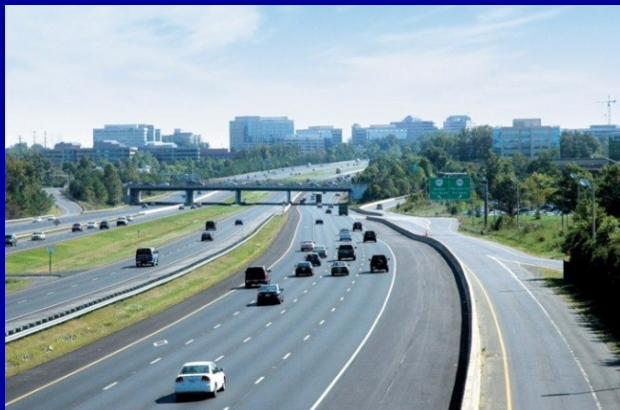
Dulles Toll Road
