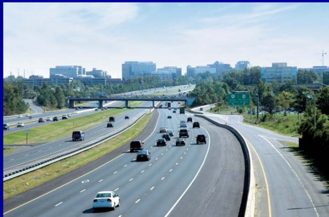
Dulles Toll Road
