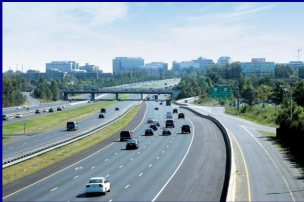
Dulles Toll Road
