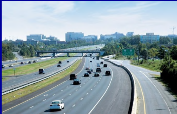
Dulles Toll Road
