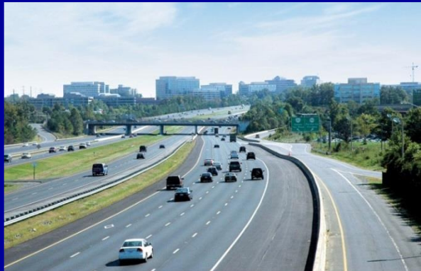
Dulles Toll Road
