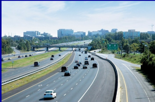
Dulles Toll Road
