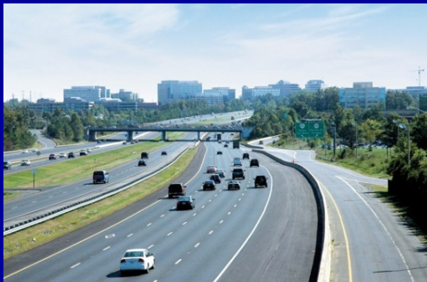
Dulles Toll Road
