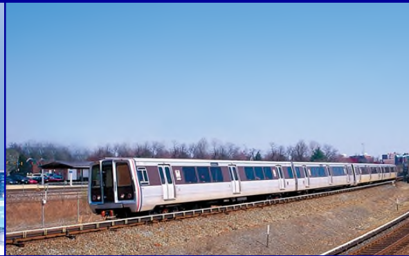
Dulles Corridor Metrorail Project
