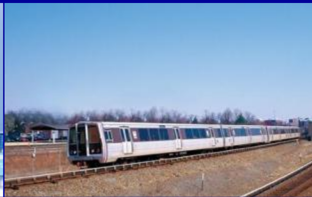
Dulles Corridor Metrorail Project
