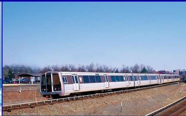
Dulles Corridor Metrorail Project
