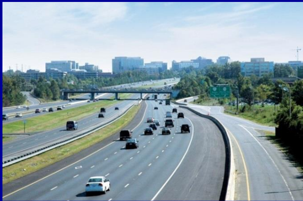
Dulles Toll Road
