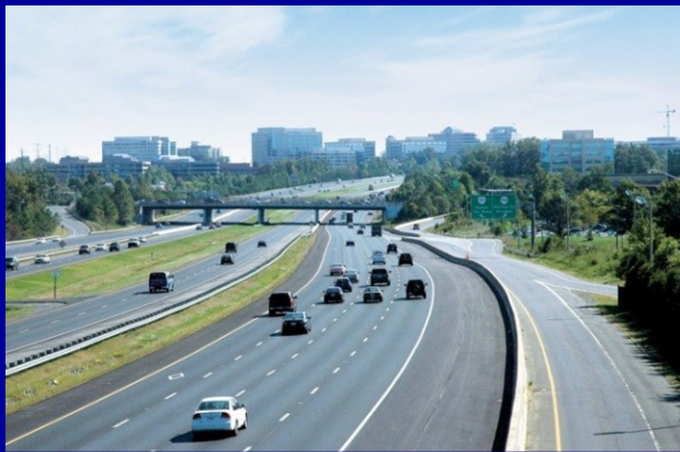
Dulles Toll Road
