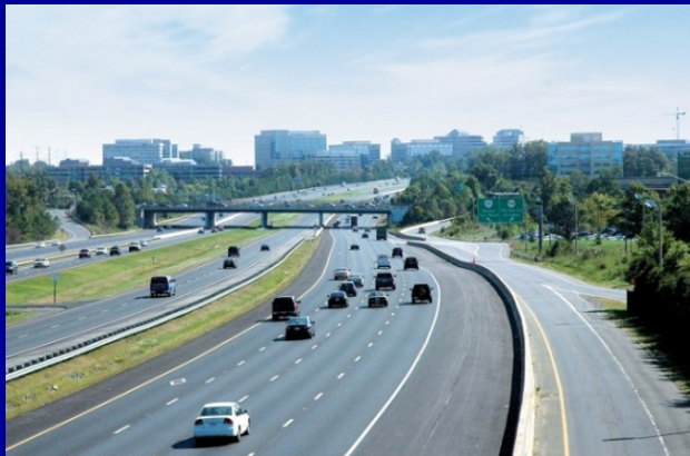
Dulles Toll Road
