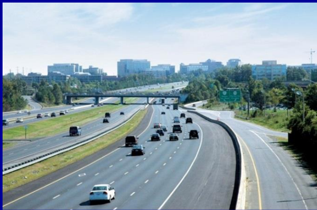
Dulles Toll Road
