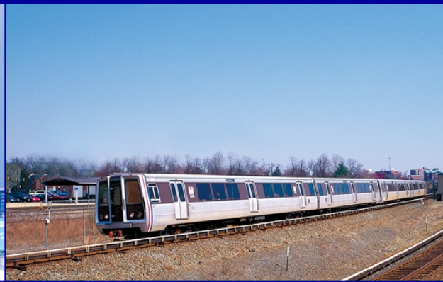
Dulles Corridor Metrorail Project
