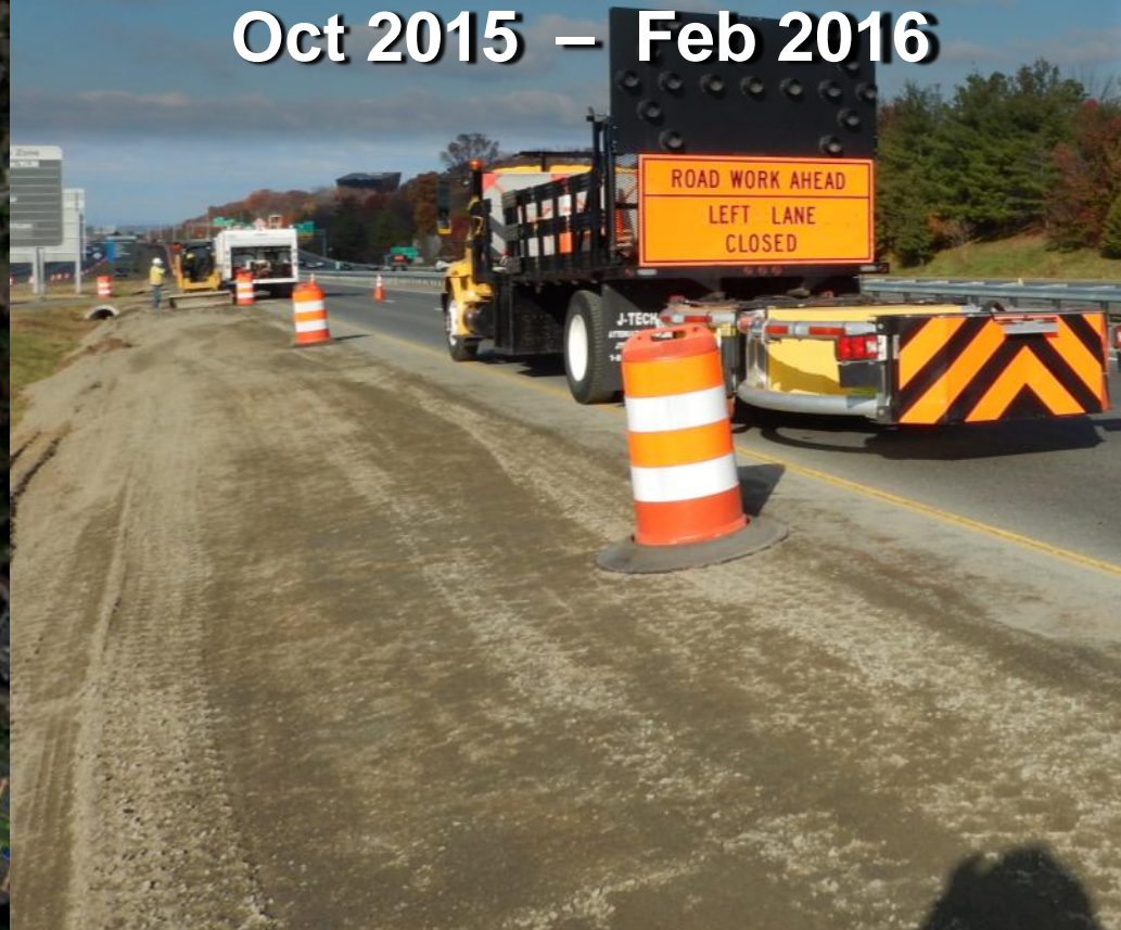
Shoulder Widening for Innovation Station
