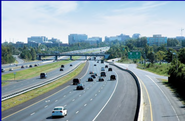
Dulles Toll Road
