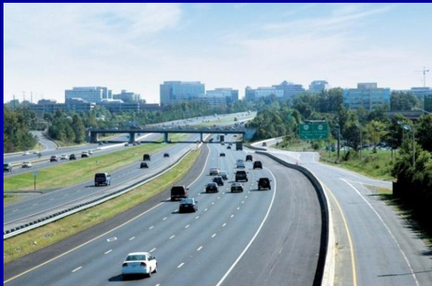
Dulles Toll Road
