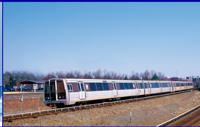
Dulles Corridor Metrorail Project
