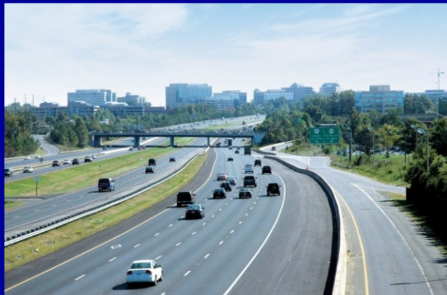
Dulles Toll Road
