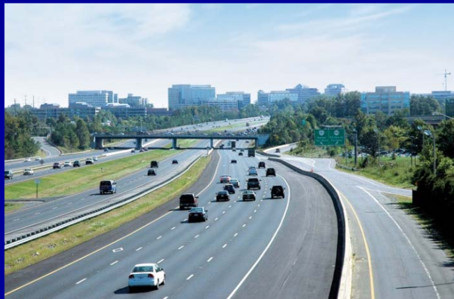
Dulles Toll Road
