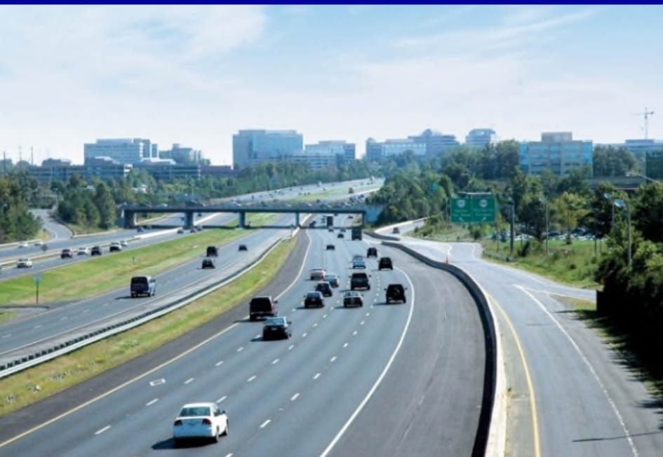
Dulles Toll Road
