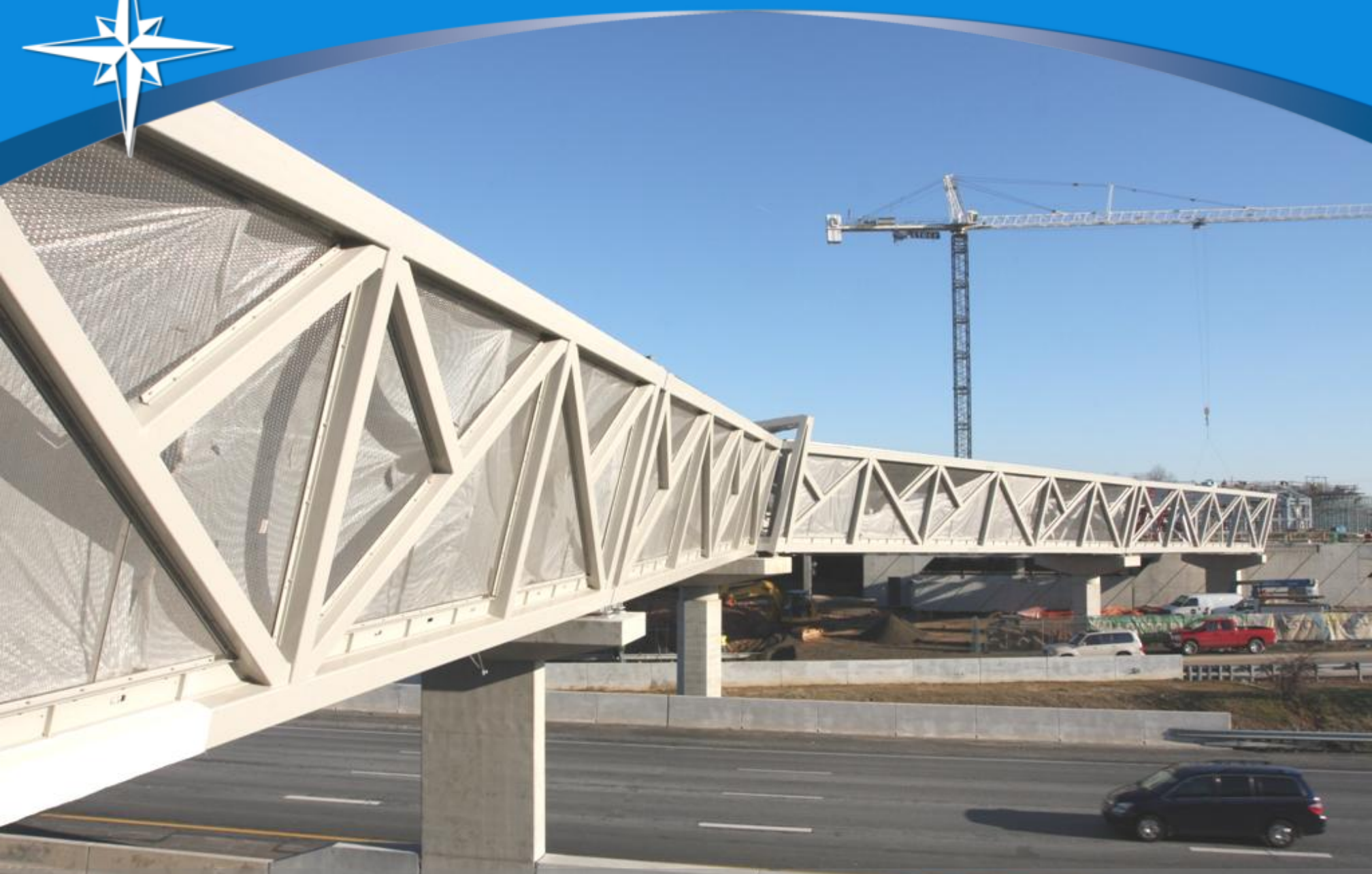
Wiehle-Reston East Station – Pedestrian Bridge
