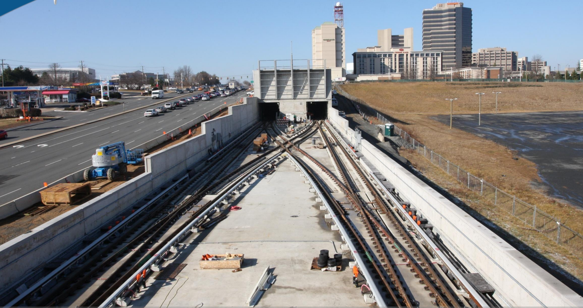
Tysons Corner Station – Double Crossover into Tunnel
