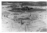
The Airport was originally designed with four runways: the main north-south runway at 6,855 feet; a northwest-southeast runway at 5,210 feet; a northeast-southwest runway at 4,892 feet; and an east-west runway at 4,100 feet.
