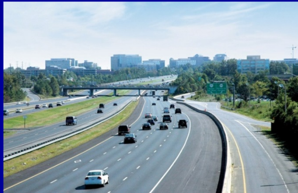
Dulles Toll Road
