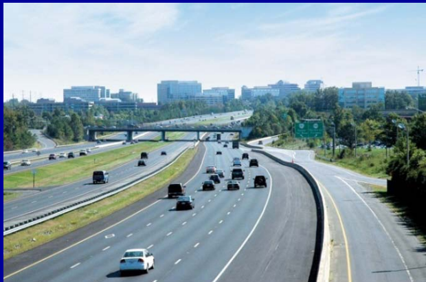
Dulles Toll Road
