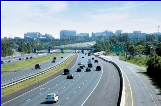
Dulles Toll Road
