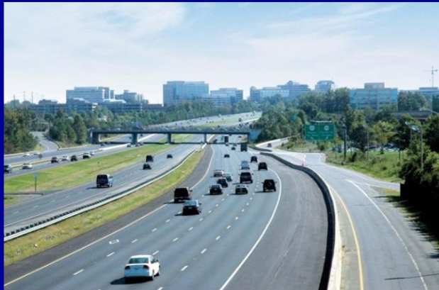
Dulles Toll Road
