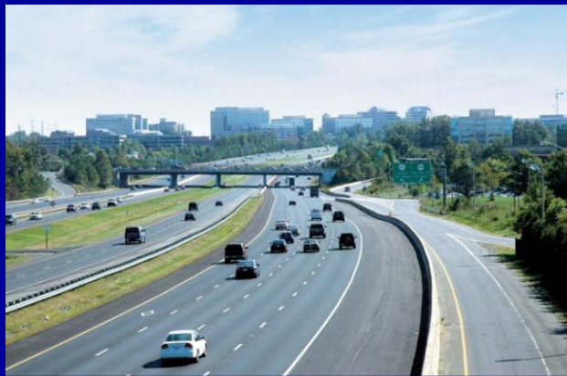
Dulles Toll Road
