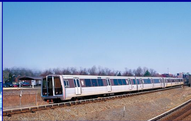
Dulles Corridor Metrorail Project
