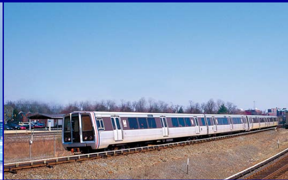
Dulles Corridor Metrorail Project
