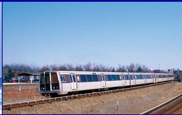
Dulles Corridor Metrorail Project
