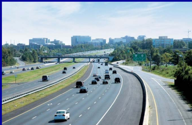
Dulles Toll Road
