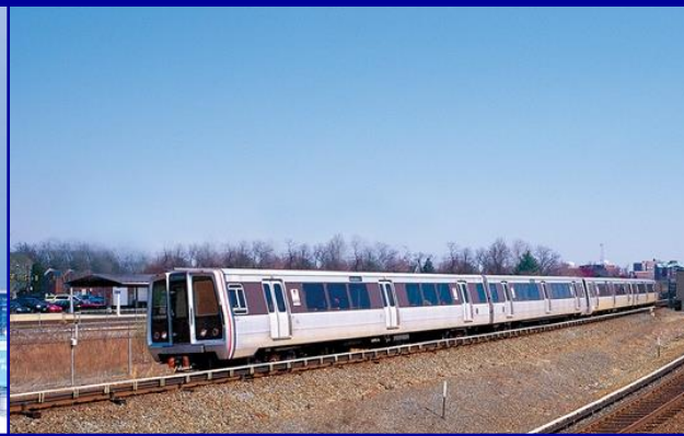
Dulles Corridor Metrorail Project
